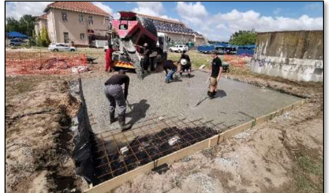
Construction of Concrete Slab
