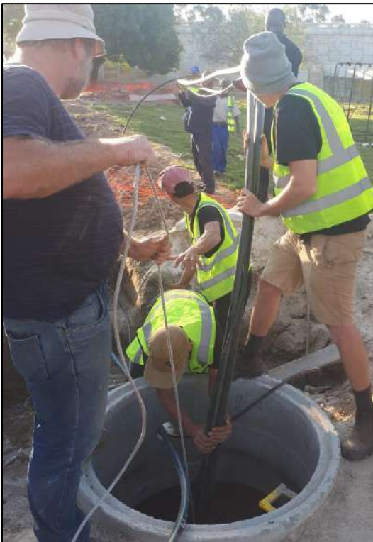
Installation of Borehole Pump
