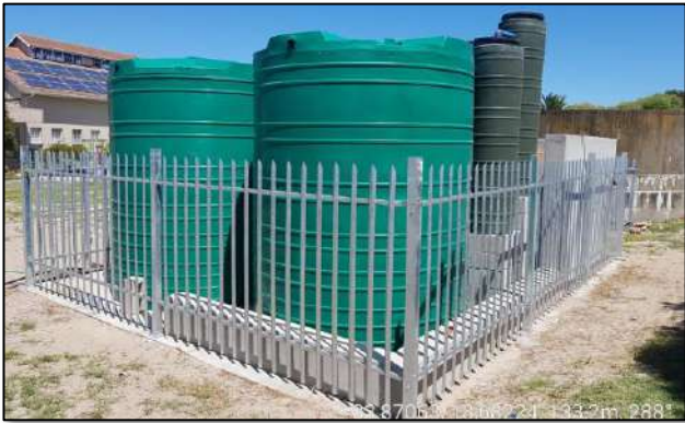
Civil Works and Water Storage Tanks
