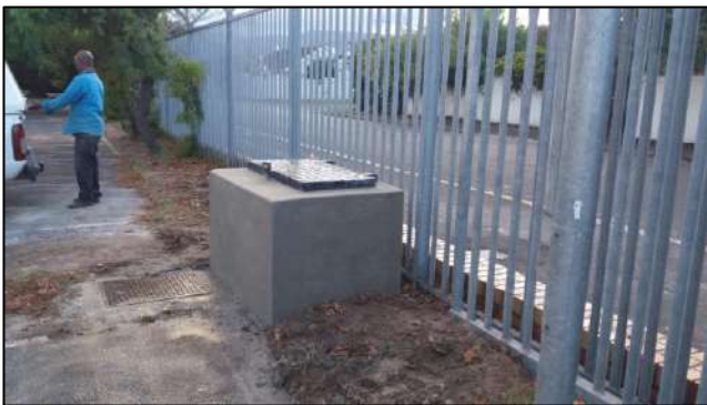
RPZ Chamber Construction
