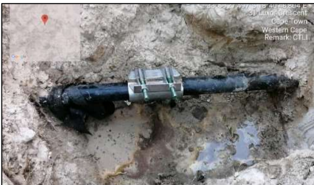
Leak Detection Repairs
