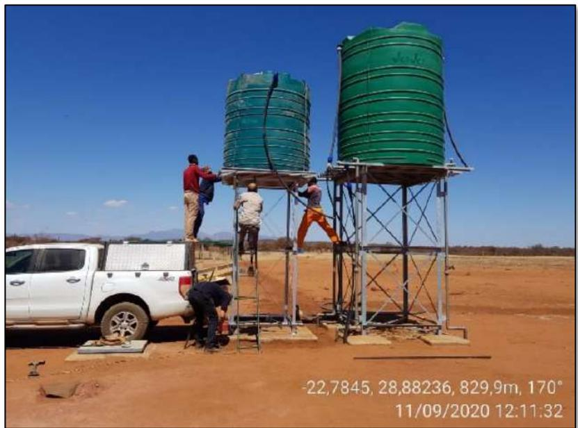
*Installed tank stands with reinforced concrete bases*
