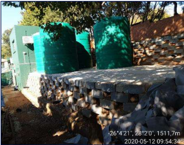
Newly constructed retaining walls and concrete slab to house the plant
