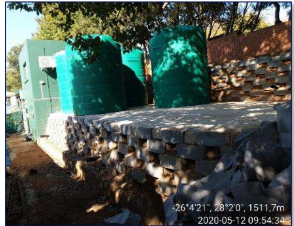
Positioning of plant filters and water storage tanks following their delivery
