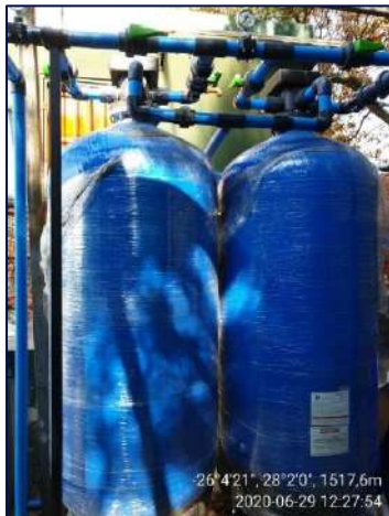
Installation of the plant filters and piping
