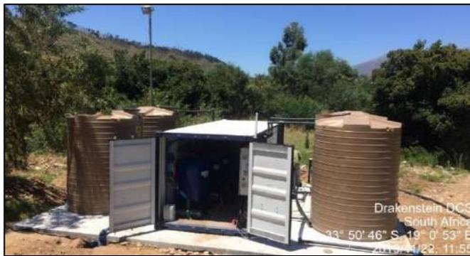
*Containerised WTW, including pre- and post-treatment water storage tanks*
