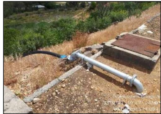
*Outlet tie-in into the existing elevated reservoir that supplies the facility with water*
