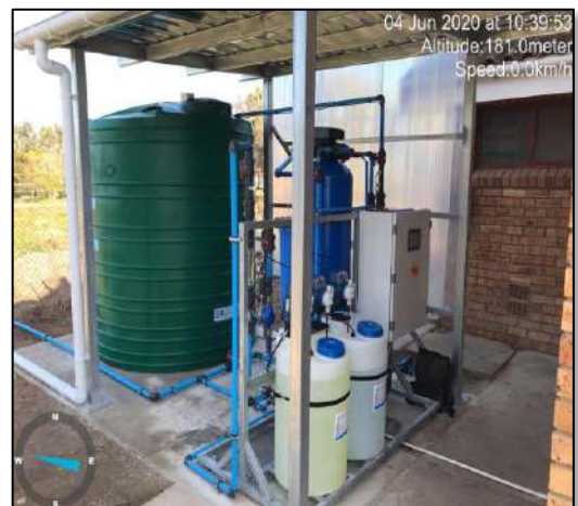
Supporting housing structure constructed for WTW
